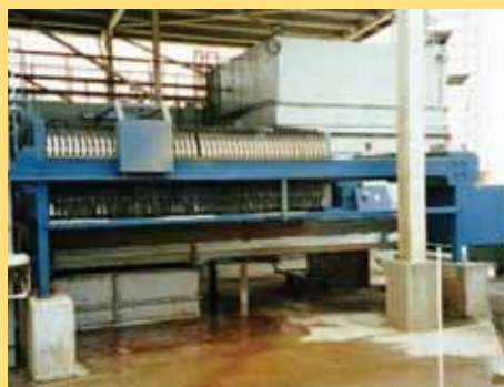
Acetylene Gas Production
